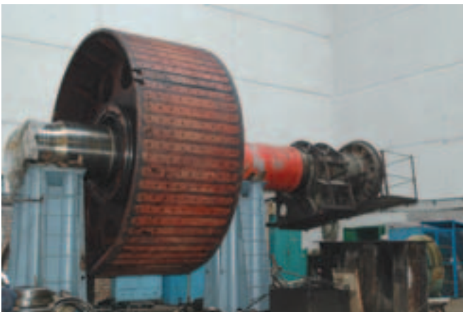
Ukraine UkrHydroEnergo Hydro Rehabilitation project
