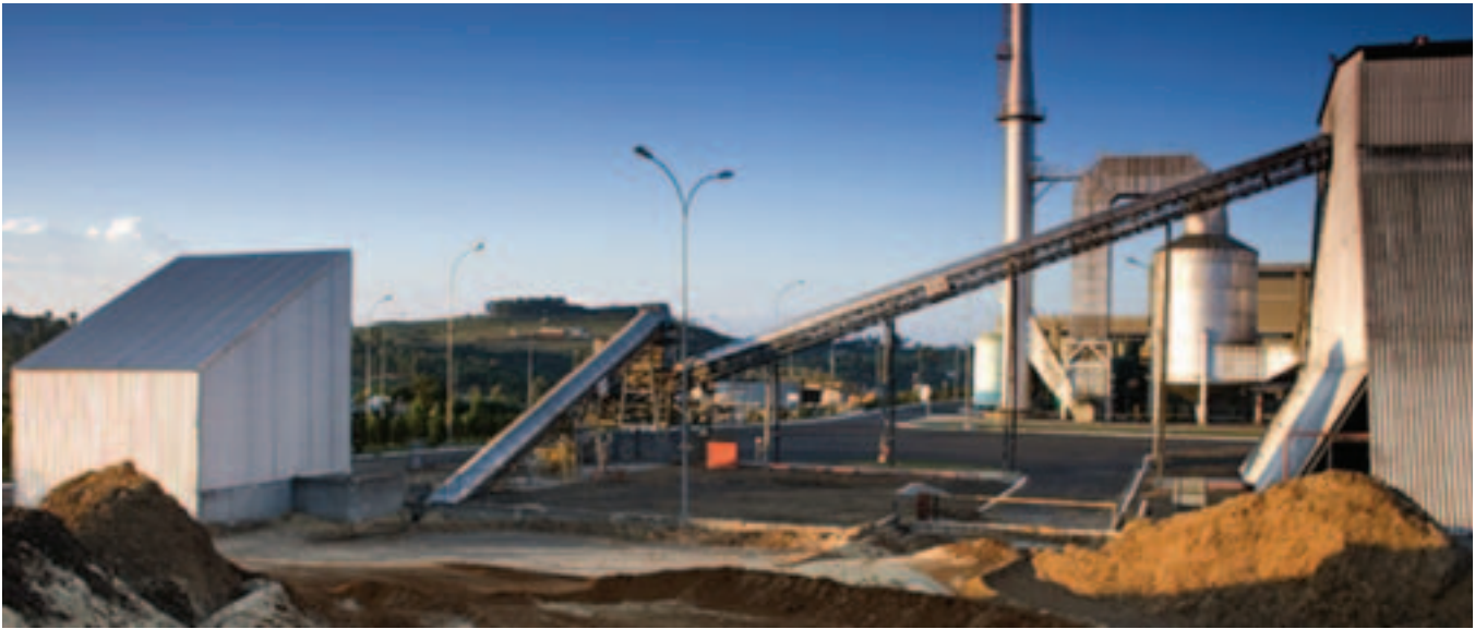
The PCF portfolio consists of 24 transactions worth approximately $181.4 million. The PCF closed its portfolio by signing its last emission reductions purchase agreement for the Brazil Lages Cogen Facility project in January 2007. The project will use wood waste from wood industry activities to generate electricity and steam.
