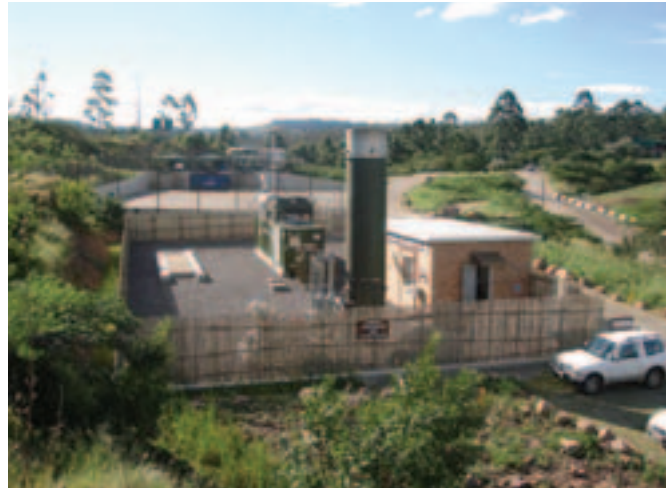
South Africa Durban Municipal Solid Waste project (PCF)
