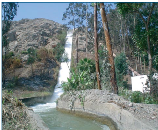
A canal and spillway at the Santa Rosa hydro project. The canal is cleaned regularly as part of the community benefits plan.
