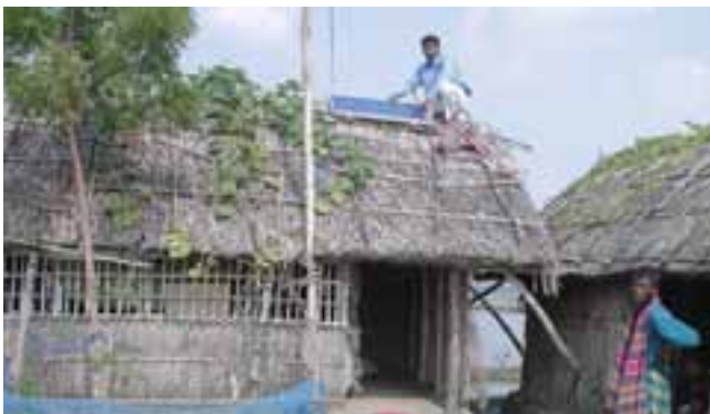
Installation of 65,000 solar home systems in Bangladesh also generates carbon credits.
