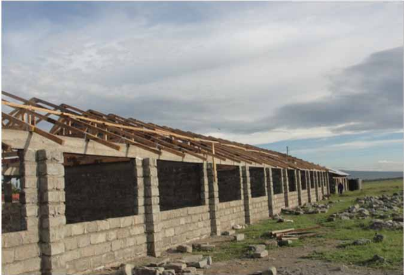
Oloirowua Primary School under construction.
