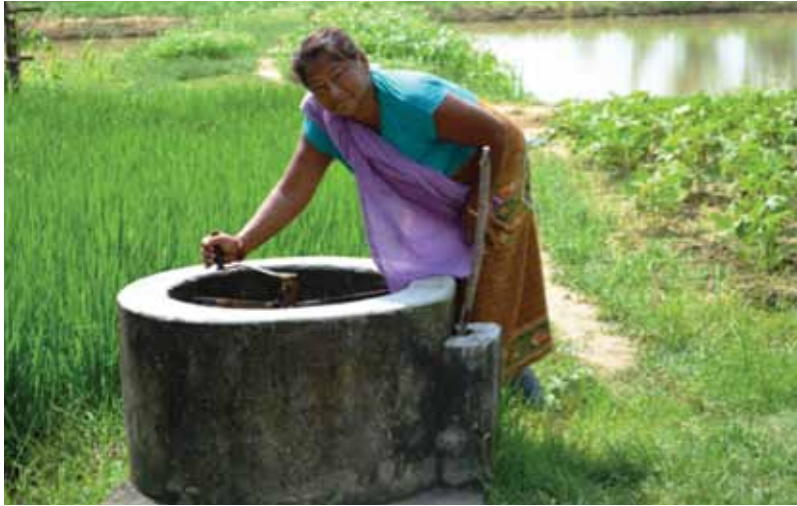
Woman churning animal waste in biodigester to create clean gas for cooking.
