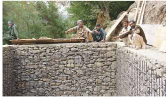
Construction of micro hydro unit by community-based organization
