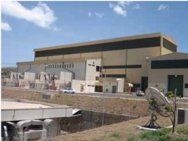
Olkaria II Geothermal Plant.
