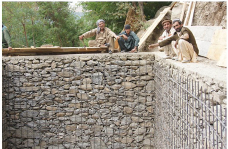
Construction of a micro hydro plant by a community-based organization.
